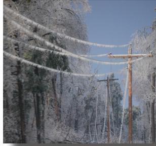
Galloping is the bouncing or bucking movement of overhead lines and can cause several problems, from temporary power interruptions to equipment damage, the collapse of power poles and downed lines.
