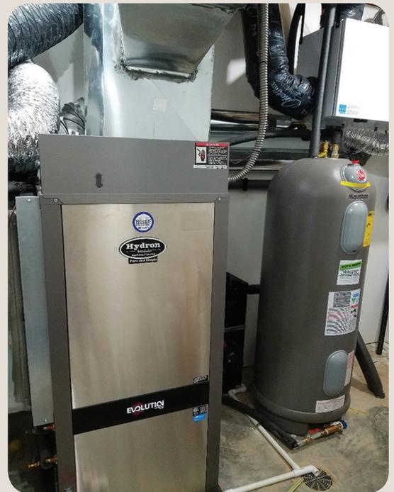
Member installed geothermal heat pump with desuperheater hot water heater.
