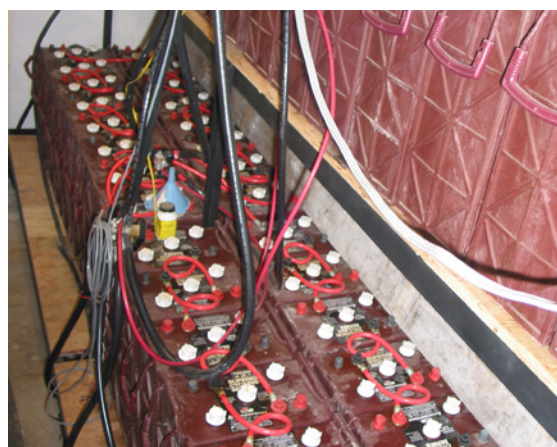
▲ A battery bank
