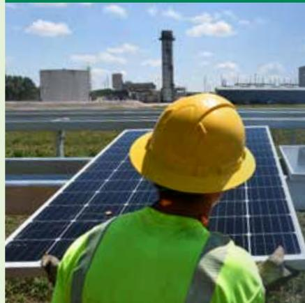
A new single-axis tracking panel is installed at Corn Belt Power Cooperative's new 150-kilowatt solar project at Wisdom Station, Spencer, Iowa. This 600-panel project replaces the space once occupied by the plant's coal pile. Photo taken by Marena Fritzler, marketing director, Corn Belt Power Cooperative. ⚡
