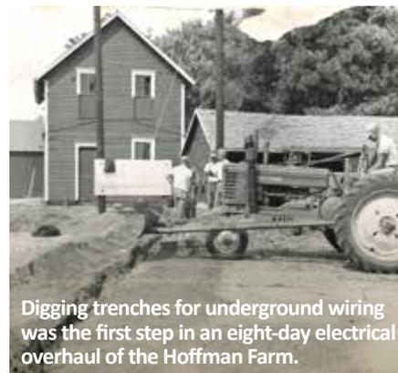
Digging trenches for underground wiring was the first step in an eight-day electrical overhaul of the Hoffman Farm.
